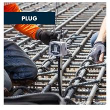
Plug the sensors into the transmitter node for wireless connectivity.
