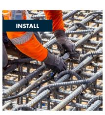
LumiCon sensors are easy to install. Simply secure the sensors to rebar with tie wraps.
